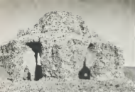
Typical fire temple has square chamber entered through four arches and crowned by dome. Entering corridor, now vaulted, kept fire from being seen by passersby. (David N. Wilber photo)
